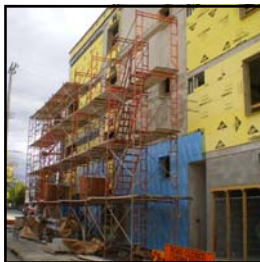
314 Booth Street during construction
